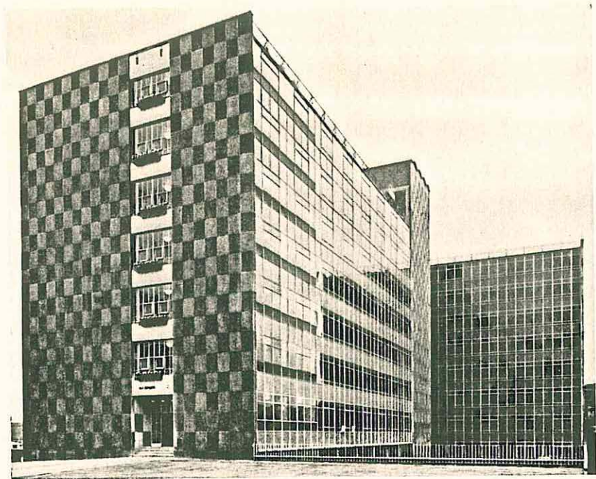
FIG. 44.—Flatted factory in Birmingham. (Photograph by courtesy of the architects, Philip Shelcker, in association with A. G. Sheppard Fiddler.)
